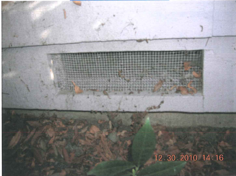
TYPICAL FOUNDATION VENT
