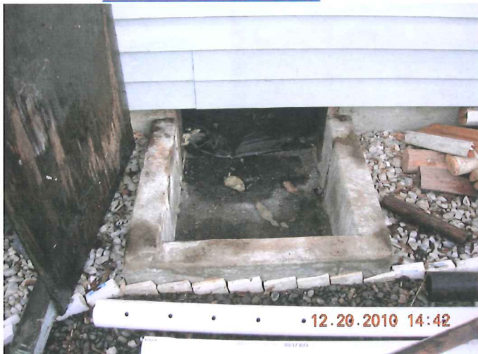
CRAWL SPACE ACCESS
