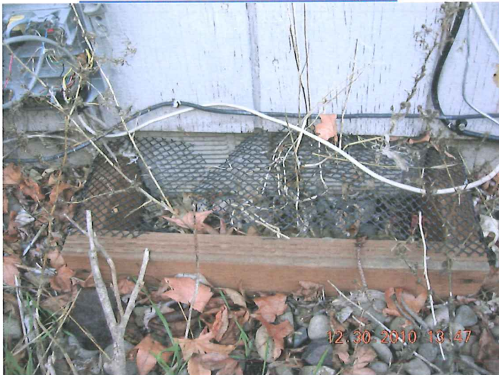
TYPICAL FOUNDATION VENT (SIX)
