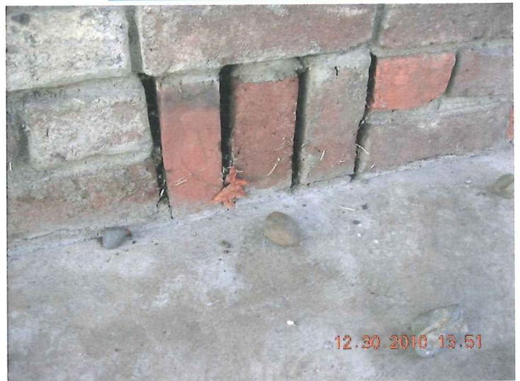
TYPICAL BRICK VENT (TWO)
