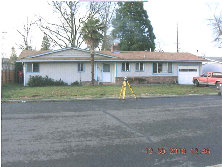
EAST FACE OF HOME
