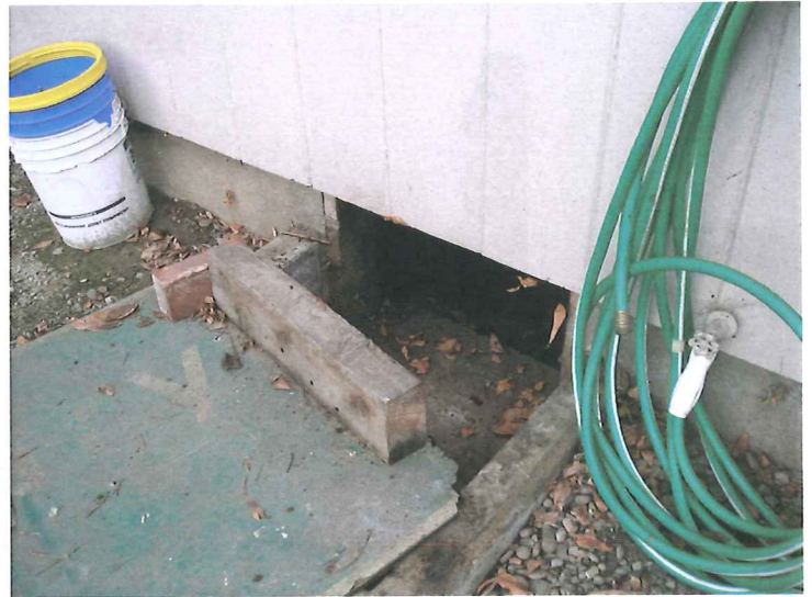
CRAWL SPACE ACCESS
