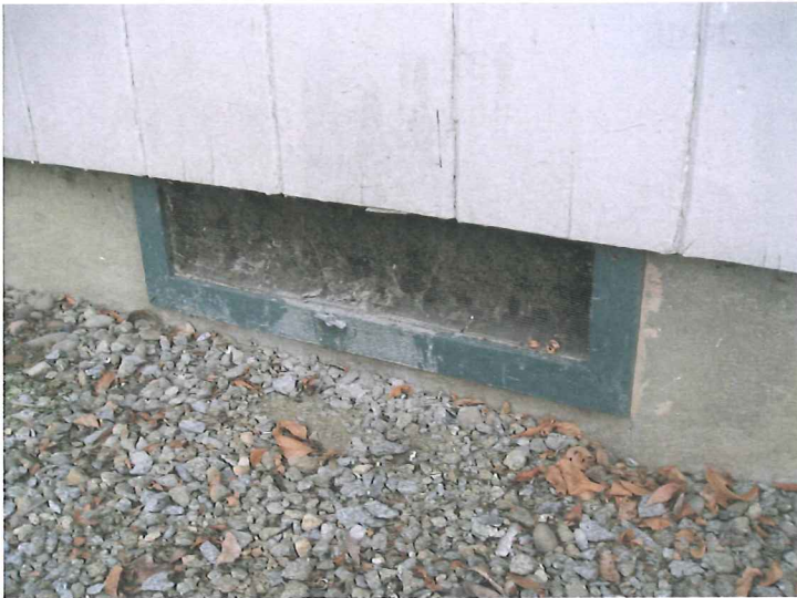
TYPICAL FOUNDATION VENT
