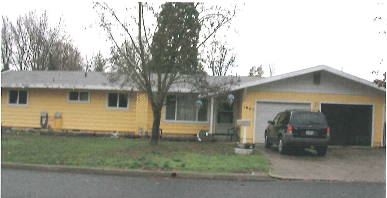
WEST FACE OF HOME
