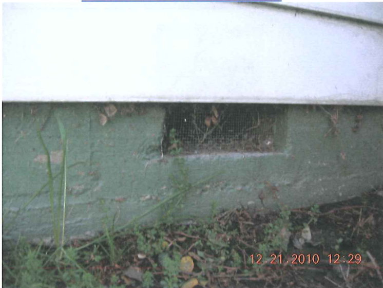
TYPICAL FOUNDATION VENT
