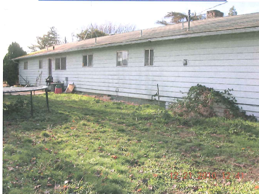
EAST FACE OF HOME (LOOKING SOUTHERLY)
