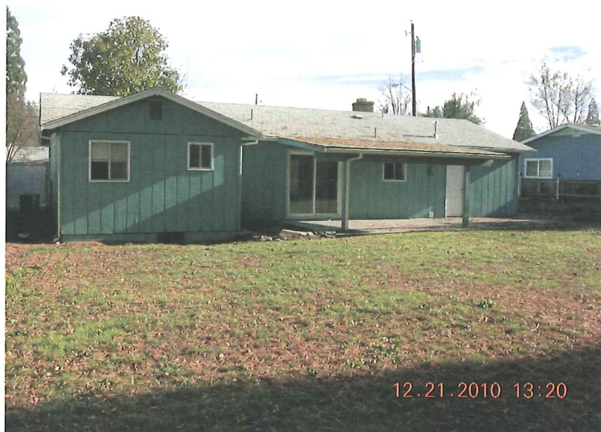
WEST FACE OF HOME
