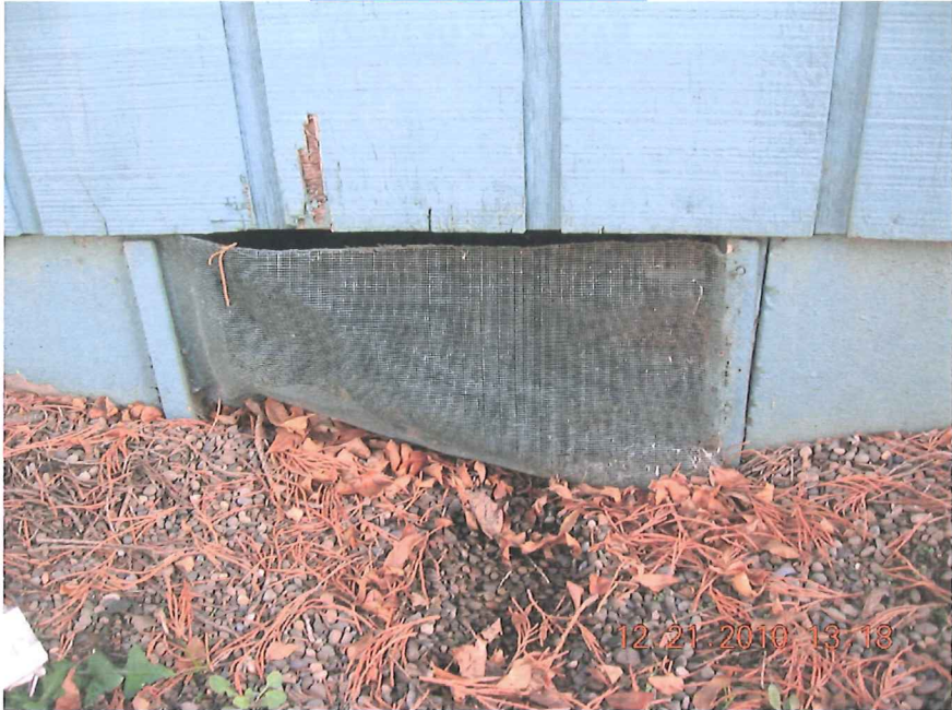
CRAWL SPACE ACCESS
