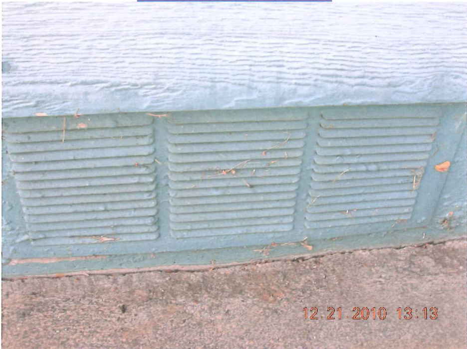
TYPICAL FOUNDATION VENT
