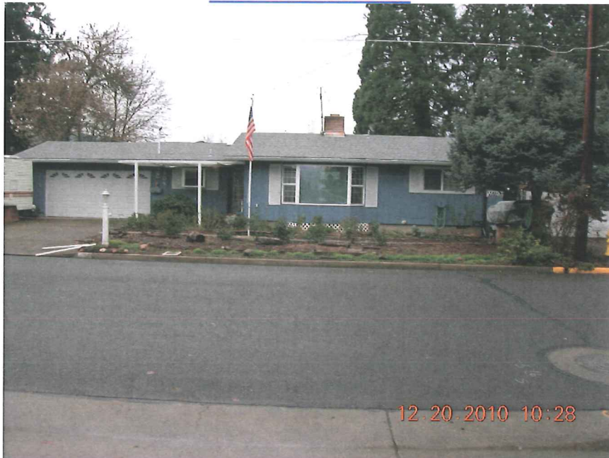
EAST FACE OF HOME
