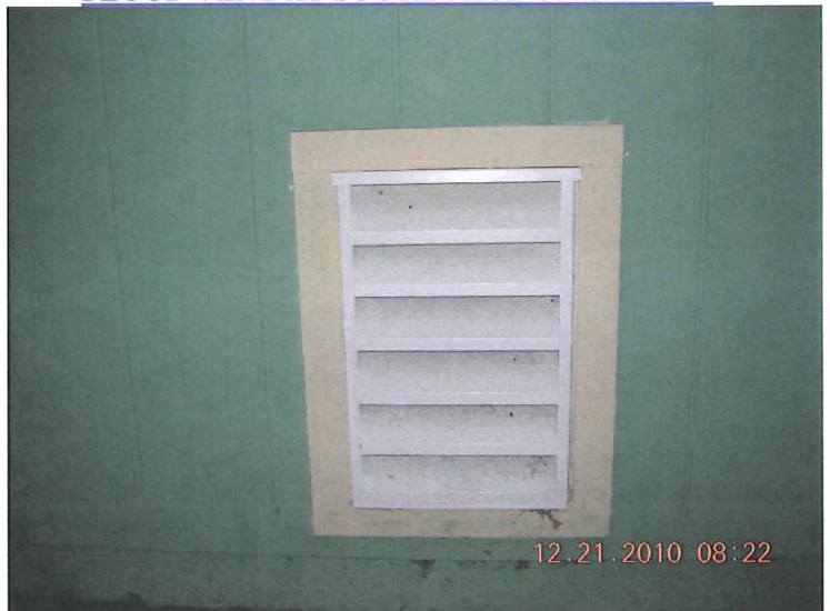
FLOOD VENT AT SOUTH FACE OF GARAGE
