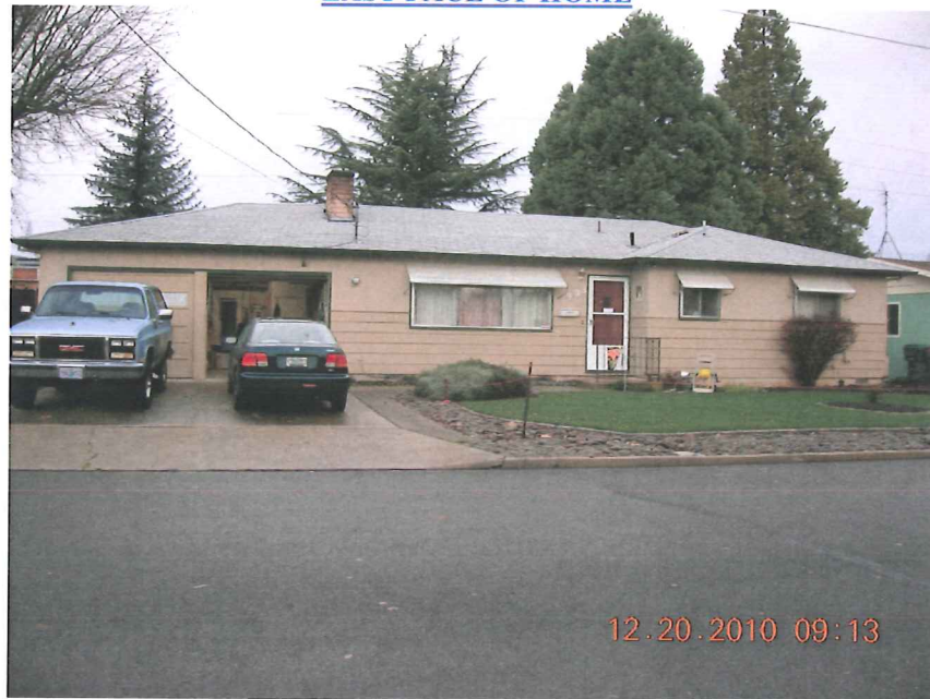
EAST FACE OF HOME
