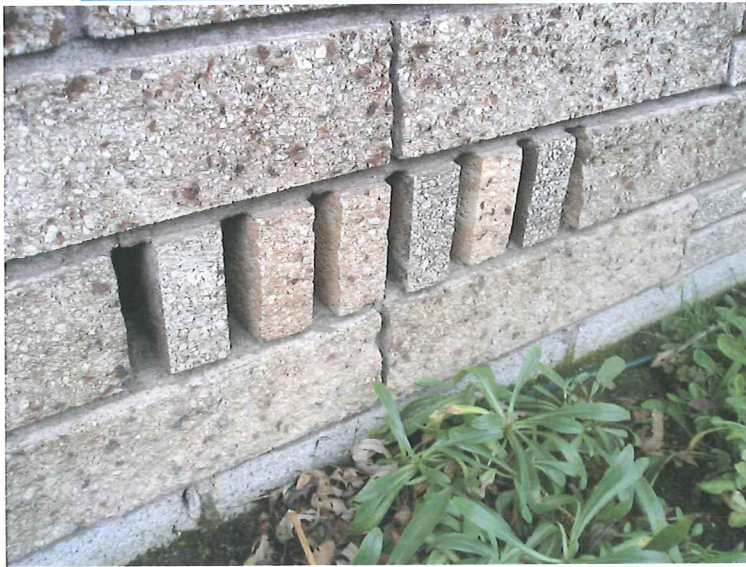
FOUNDATION VENT (2 TOTAL AT 1" X 5")
