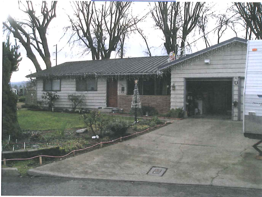
EAST FACE OF HOME
