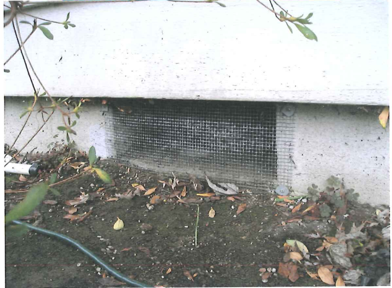
FOUNDATION VENT (8 TOTAL AT 18" X 8")
