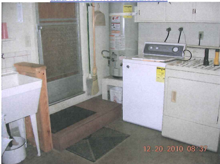
ELEVATED WATER HEATER
