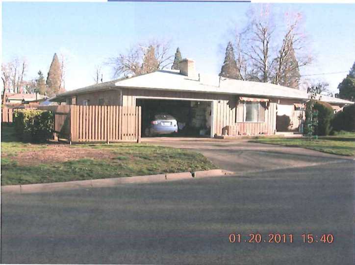
WEST FACE OF HOME
