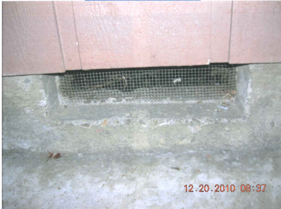
TYPICAL FOUNDATION VENT
