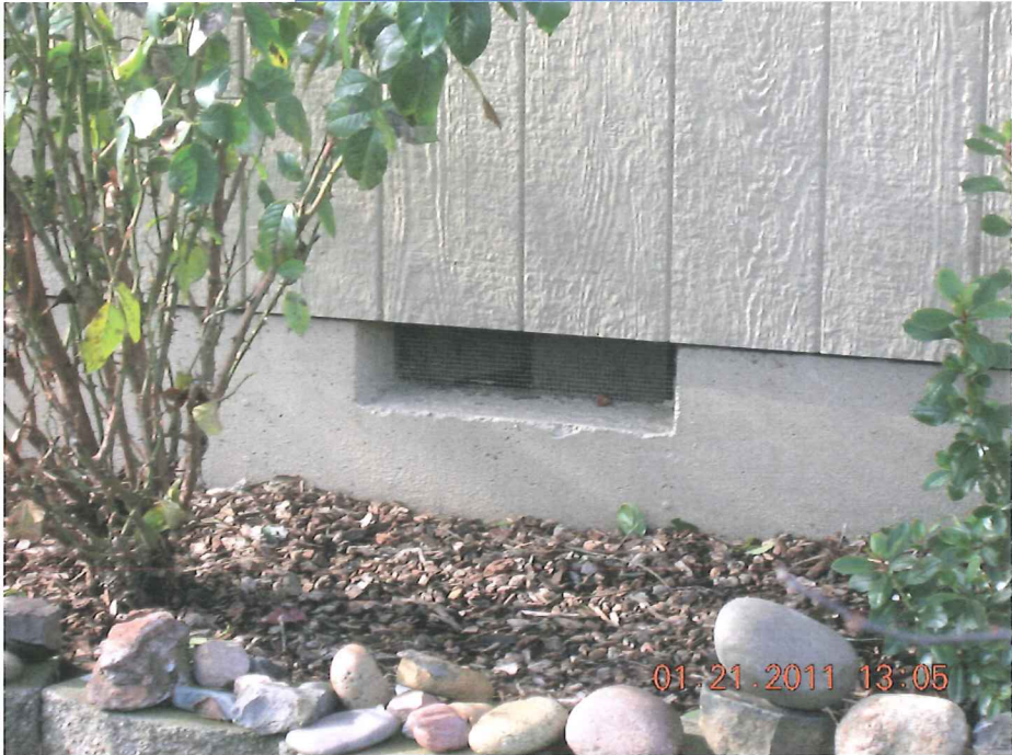
TYPICAL FOUNDATION VENT
