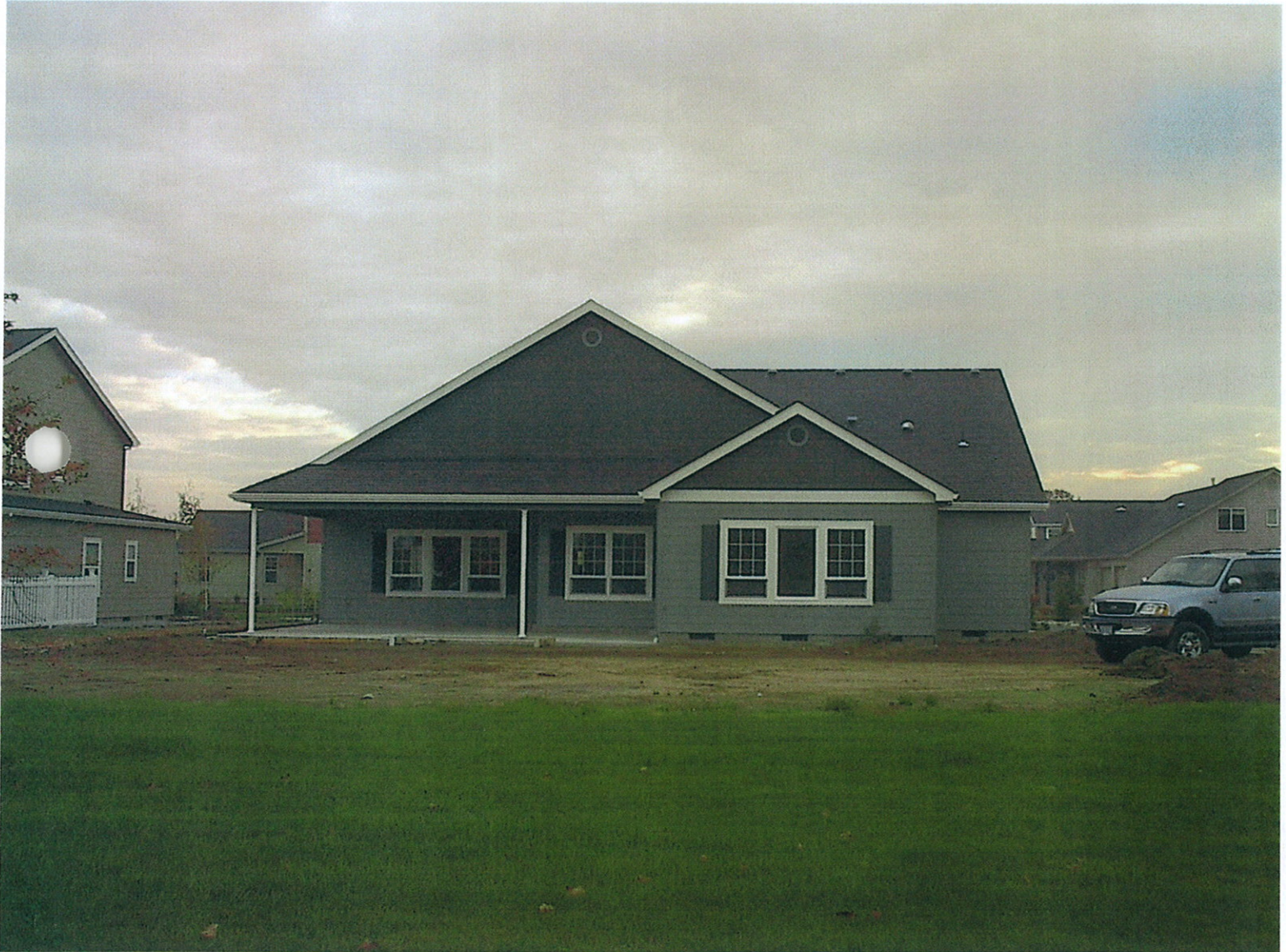
REAR VIEW (LOOKING EAST) 10/29/2007
