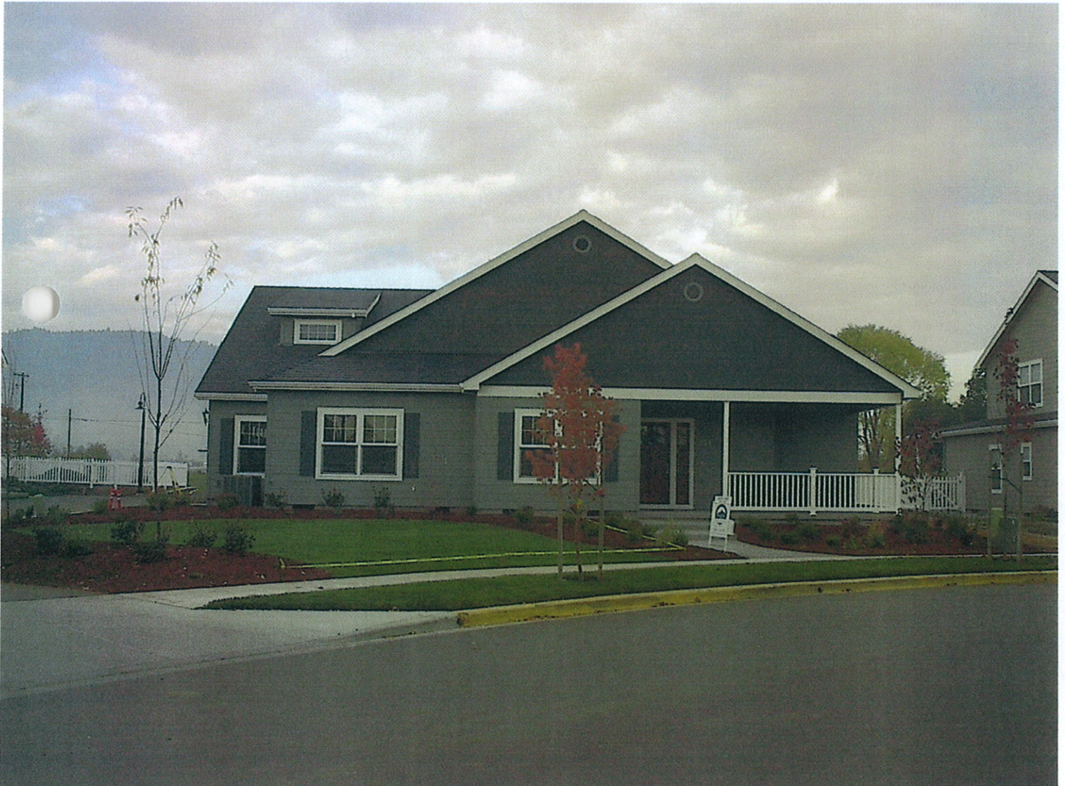
FRONT VIEW (LOOKING WEST) 10/29/2007
