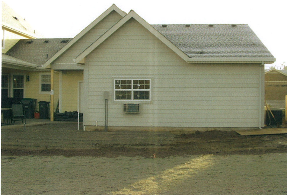
02/02/07 REAR VIEW WITH ADDITION
