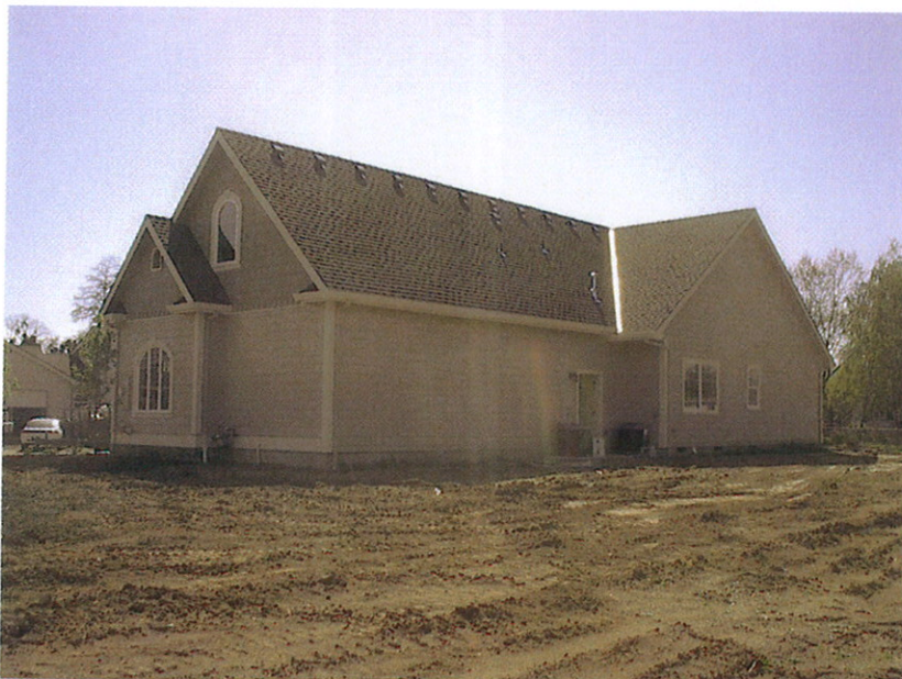
(REAR OF HOUSE LOOKING FROM NORTHWEST)
