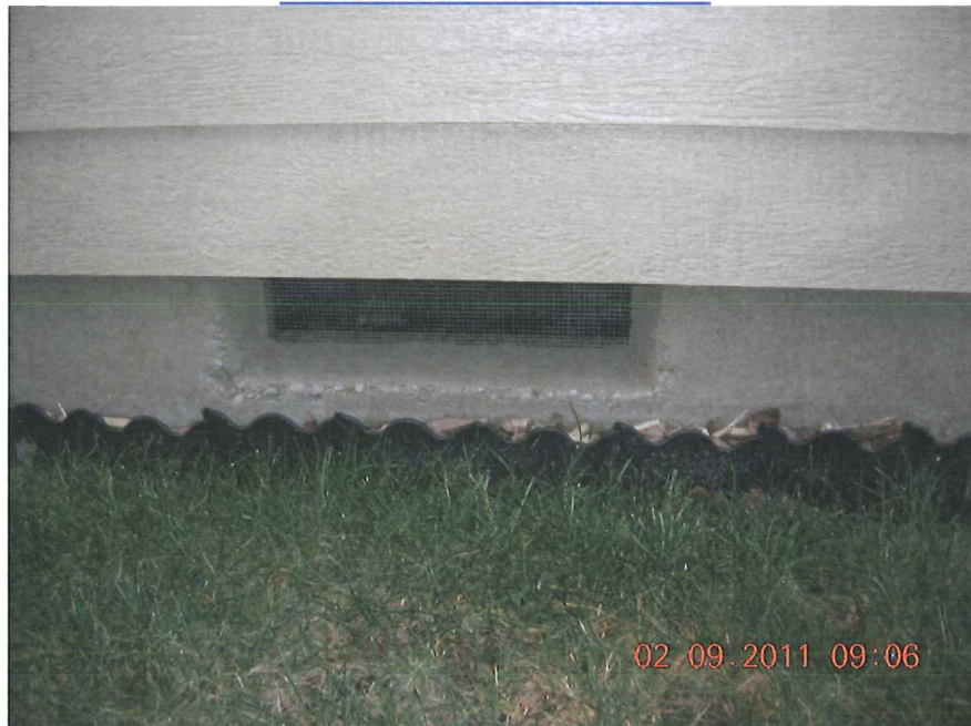
TYPICAL FOUNDATION VENT
