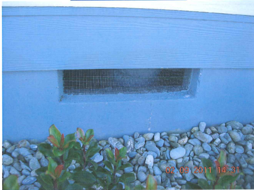
TYPICAL FOUNDATION VENT
