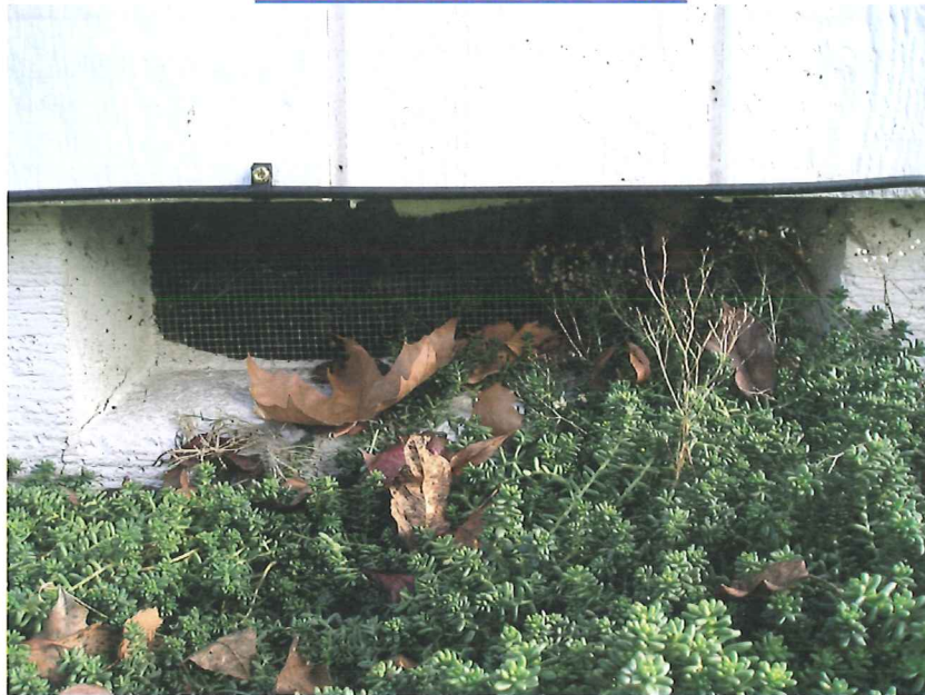
TYPICAL FOUNDATION VENT
