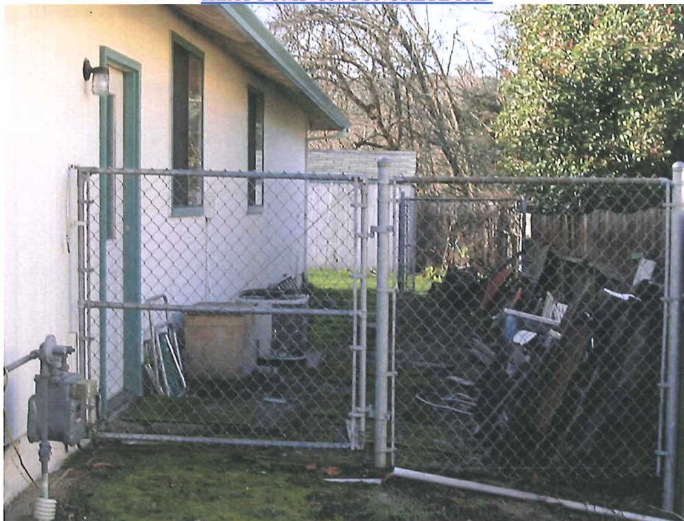
HEAT PUMP ON CONCRETE PAD
