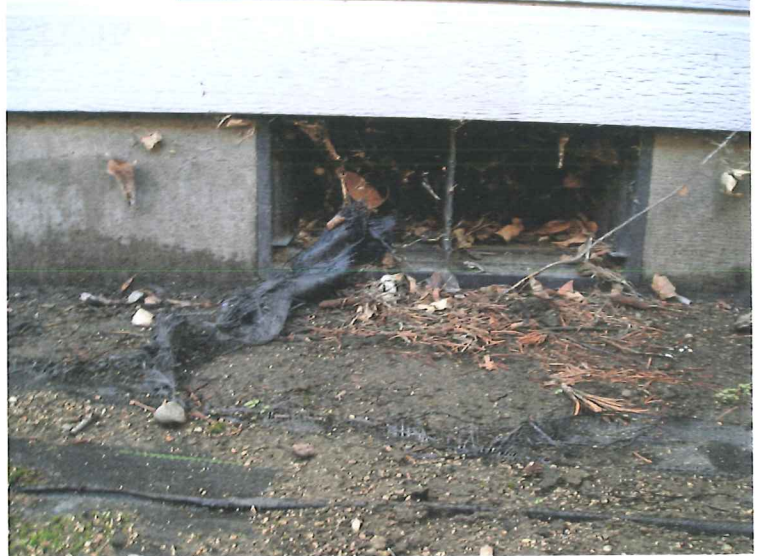
TYPICAL FOUNDATION VENT
