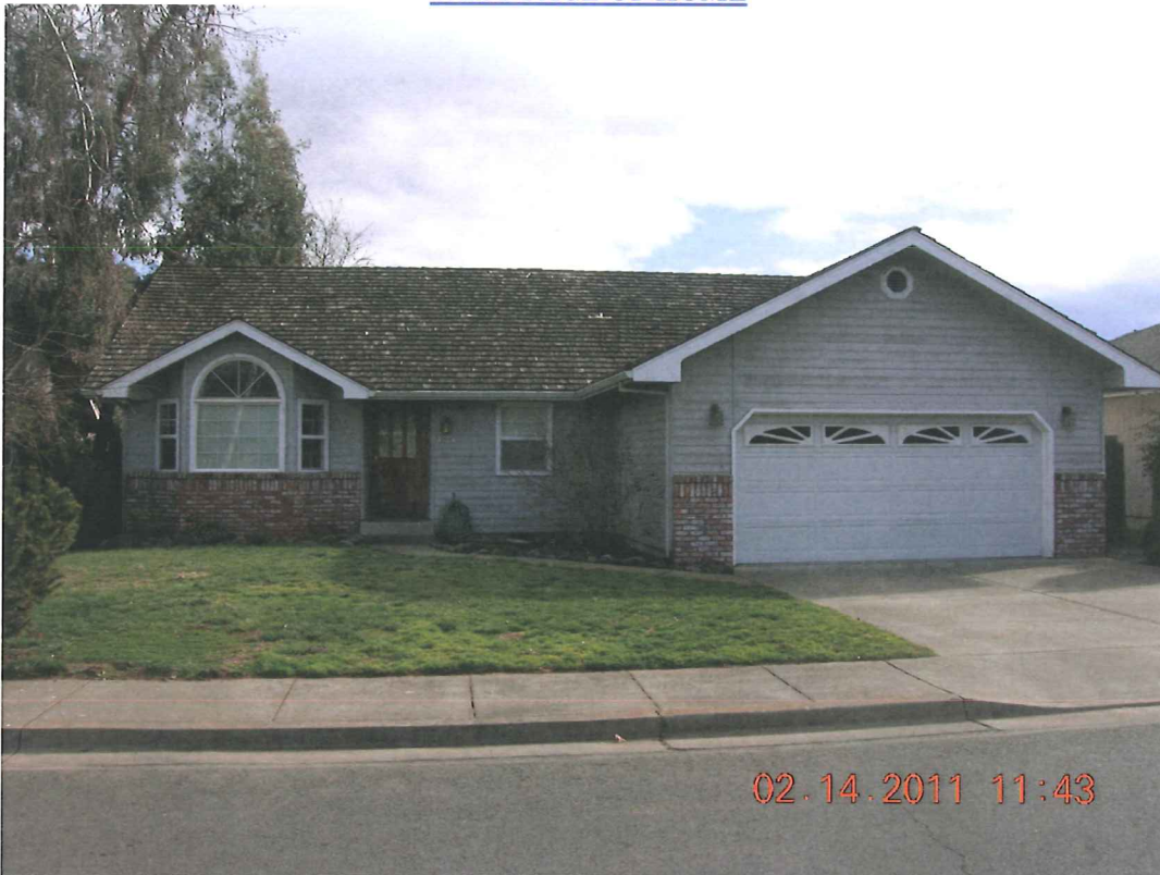
WEST FACE OF HOME
