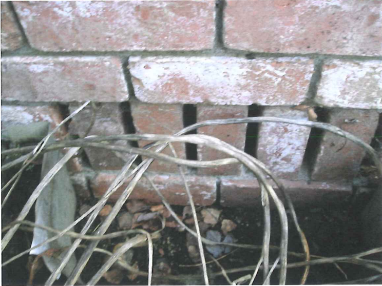
FOUNDATION VENT (VERTICAL OPEININGS IN BRICK)
