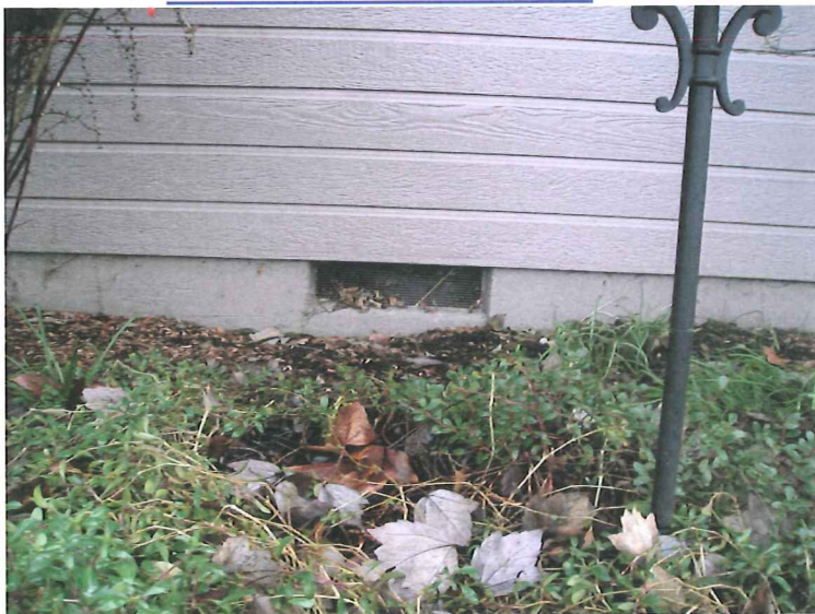
TYPICAL FOUNDATION VENT
