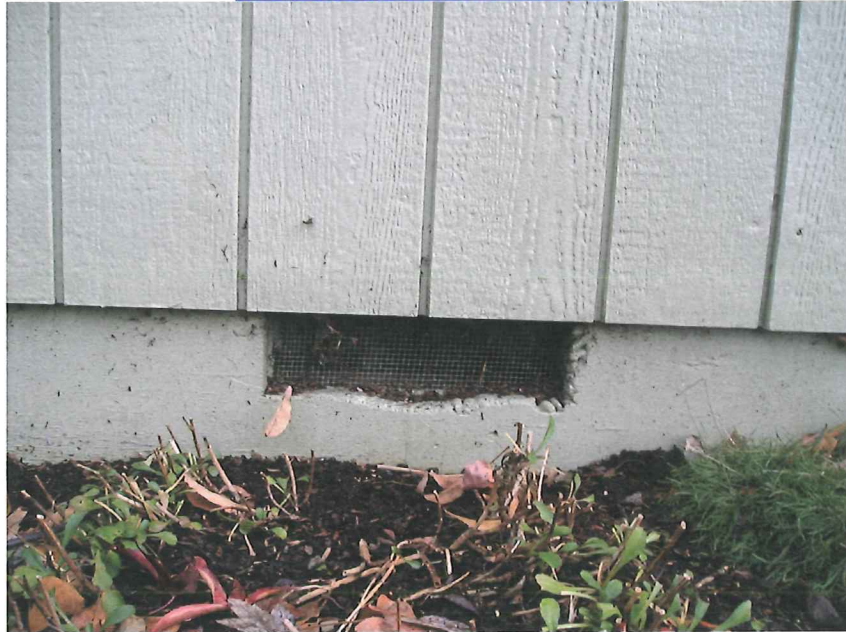
TYPICAL FOUNDATION VENT
