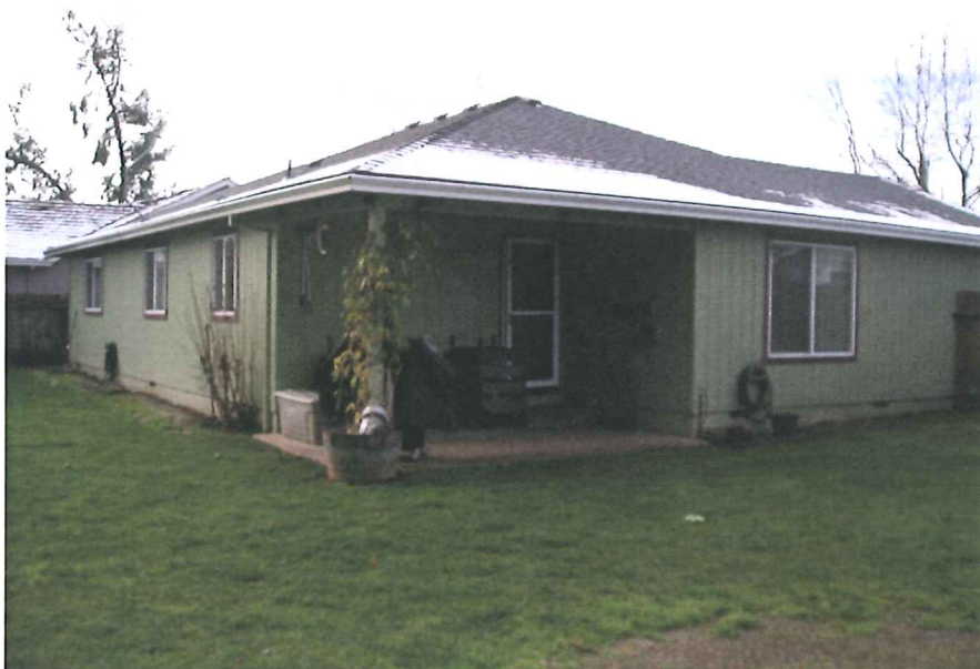
NORTHERLY & EASTERLY FACE OF HOME (LOOKING SOUTHERLY)
