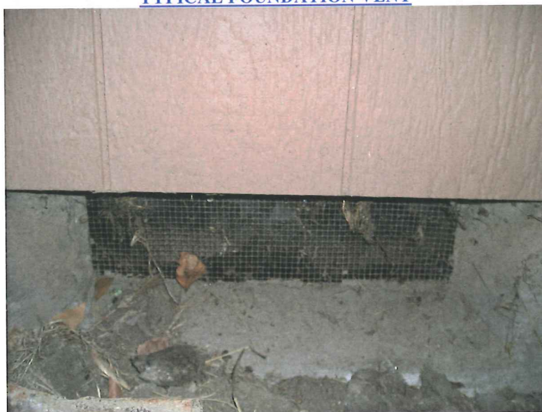
TYPICAL FOUNDATION VENT
