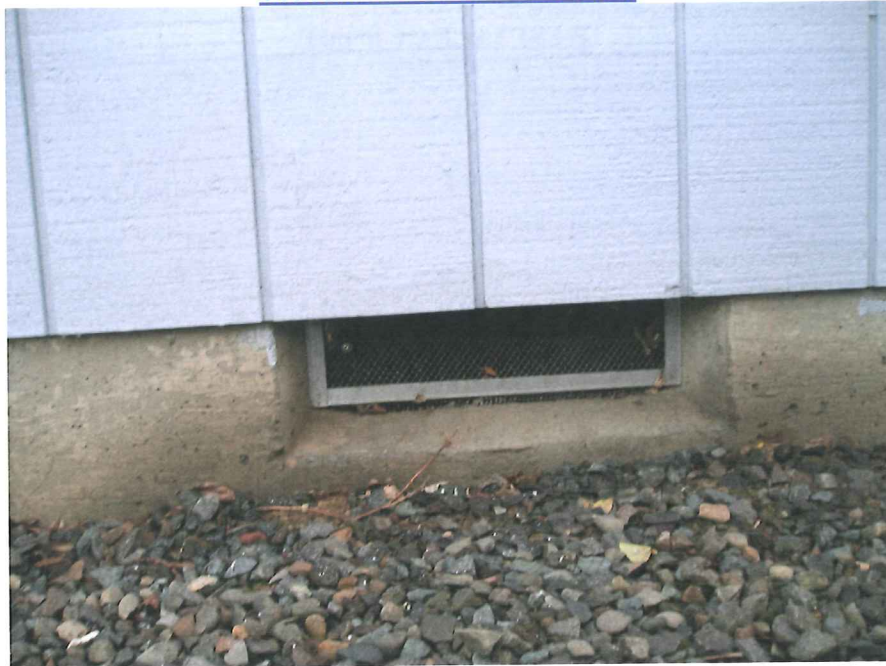
TYPICAL FOUNDATION VENT
