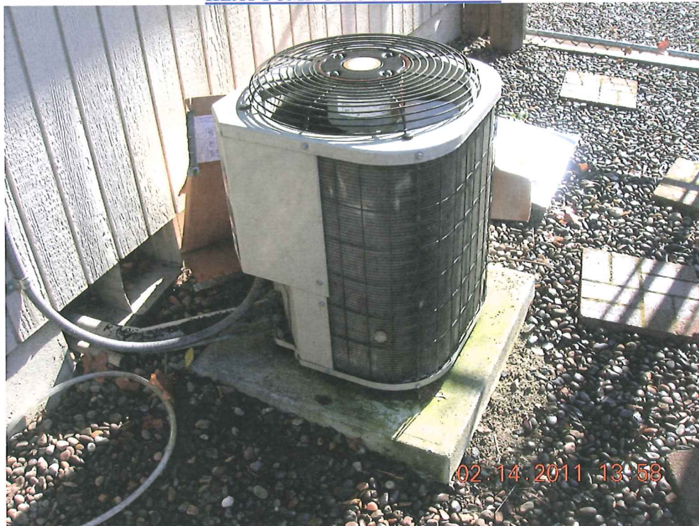
HEAT PUMP ON CONCRETE PAD
