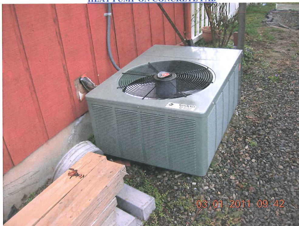
HEAT PUMP ON CONCRETE PAD
