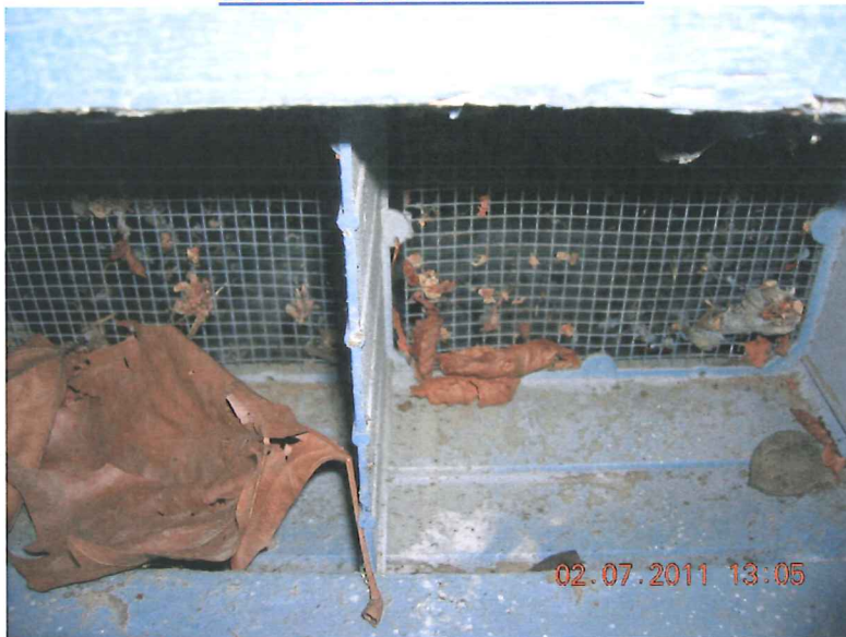
TYPICAL FOUNDATION VENT
