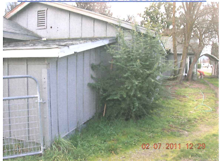
LOOKING SOUTHERLY AT WEST FACE OF HOME
