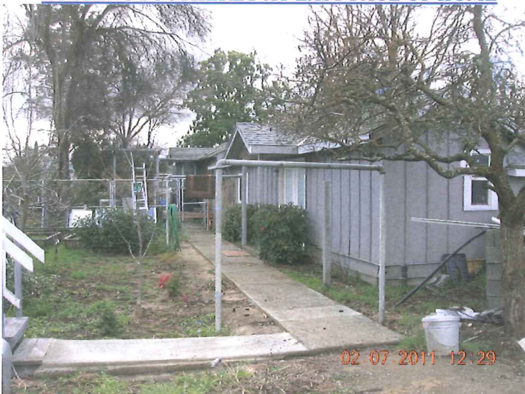
LOOKING SOUTHERLY AT EAST FACE OF HOME
