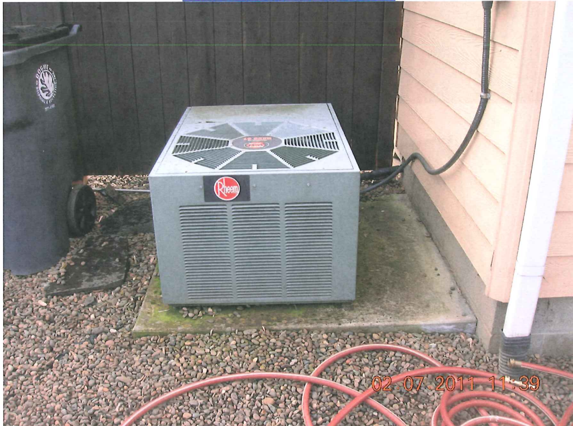
HEAT PUMP ON CONCRETE PAD
