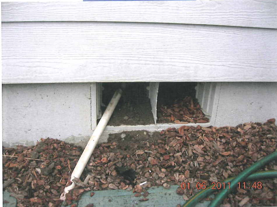
TYPICAL FOUNDATION VENT
