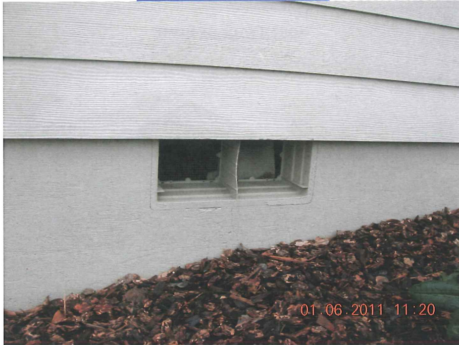
TYPICAL FOUNDATION VENT
