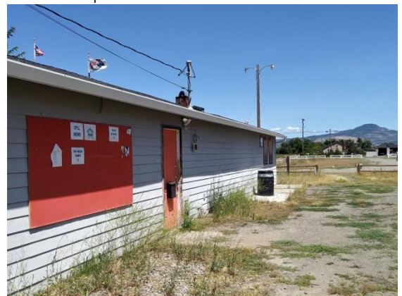
Concession stand electricity.
