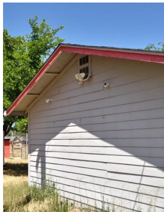
West exterior side with security cameras and lighting.
