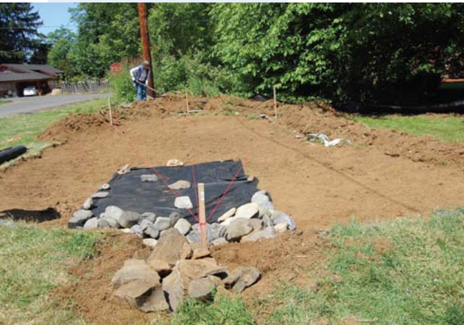
Figure 19: Grading is made simpler by using four stakes, one at the inflow point and three at the opposite or lower end of the rain garden—including, most importantly, the outflow point. (Photo: Robert Emanuel, OSU)
