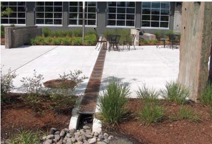
Figure 12: Trench drain through a sidewalk at a building in Portland. (Photo: Derek Godwin, OSU)
