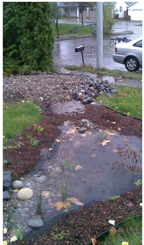
Figure 17: A rain garden in Gresham, Oregon, fills with rain. Note the use of rocks at the outflow point near top. (Photo: City of Gresham)
