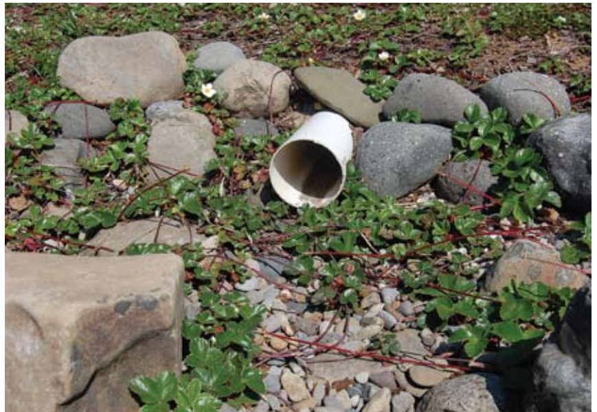
Figure 23: The point where water enters a rain garden should be well armored with rock and plants (beach strawberries here) to prevent erosion. (Photo: Robert Emanuel, OSU)
