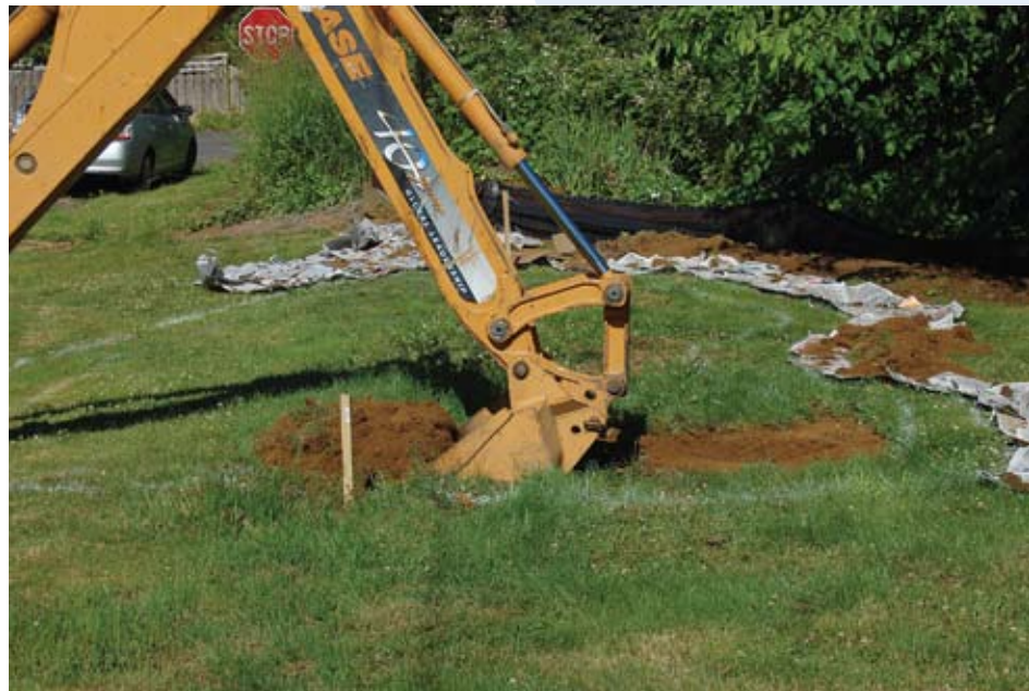
Figure 18: Excavator is located outside of the rain garden in order to make sure the machine does not compact soil in the rain garden. (Photo: Robert Emanuel, OSU)
