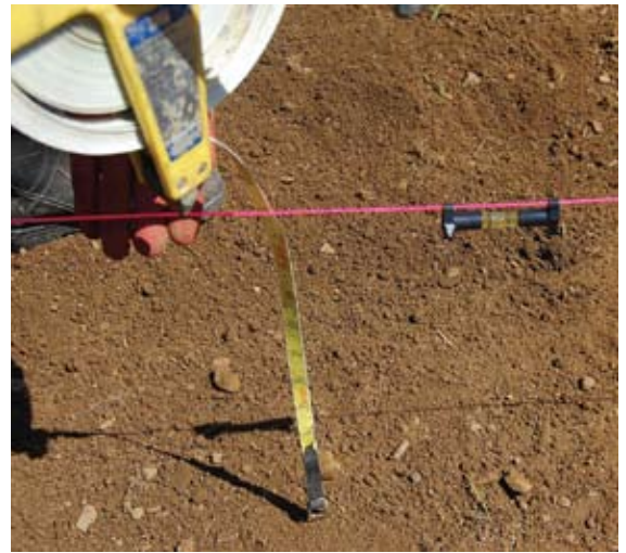
Figure 20: Using a combination of a line level and a measuring tape allows you to grade the base of the garden so that water will not pool in a particular location but will spread across the entire surface as evenly as possible. (Photo: Robert Emanuel, OSU)
