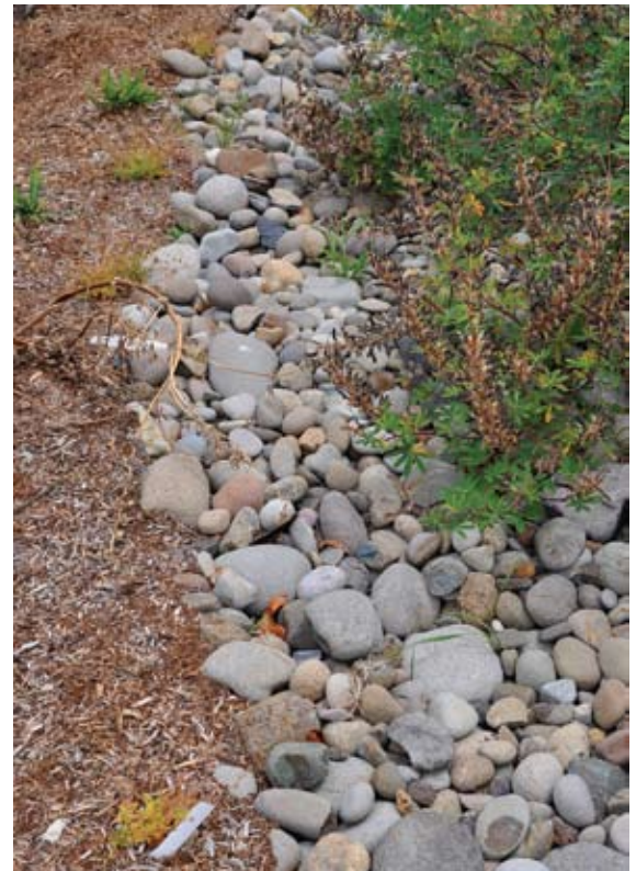
Figure 11: Using a rock-lined trench to convey water across a walkway (Photo: Portland Bureau of Environmental Services [BES])
